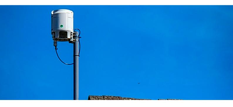
MultiHaul TG N366 distribution nodes were chosen as they feature 360-degree coverage and multiple client node options to fit a variety of deployment requirements. The N366 also provides 16 Gbps of total capacity and is installed on the roof of a centrally-located building in the area, as it has a line of sight to dozens of nearby apartment homes (see diagram below). Each home is supplied with a MultiHaul TG T260 or T265 terminal unit, which is connected to a router inside the home.
