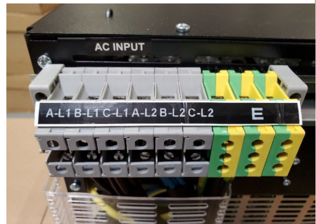
Figure 6: AC Termination
