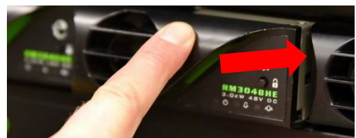
Figure 14: Inserting a Rectifier
