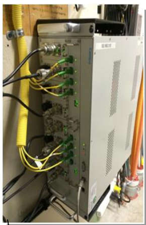
ComFlex MU 8 RFUs and 7 optical links to RU
