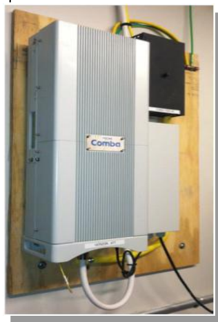
Low Power ComFlex RU 30dBm Output Power
