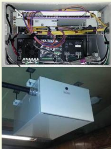
Alpha's Ceiling Mount Backup Power Solution at an underground subway station in NYC
